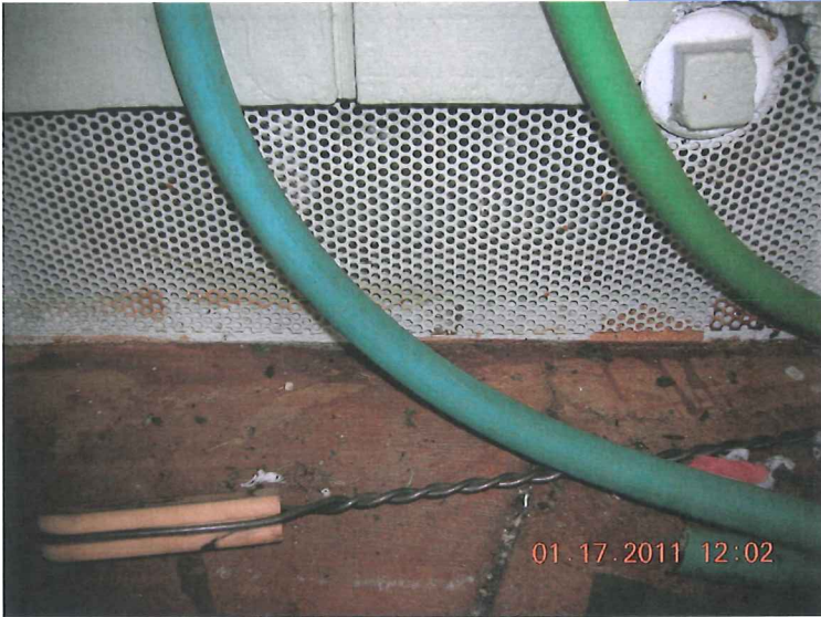
TYPICAL FOUNDATION VENT
