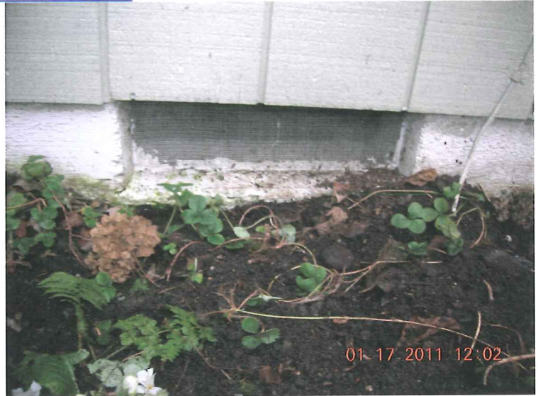
TYPICAL FOUNDATION VENT
