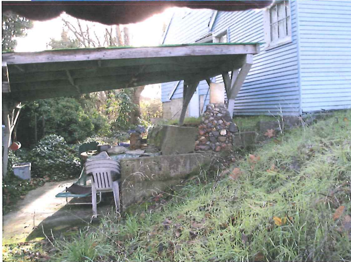
CARPORT AT NORTHERLY SIDE OF GARAGE
