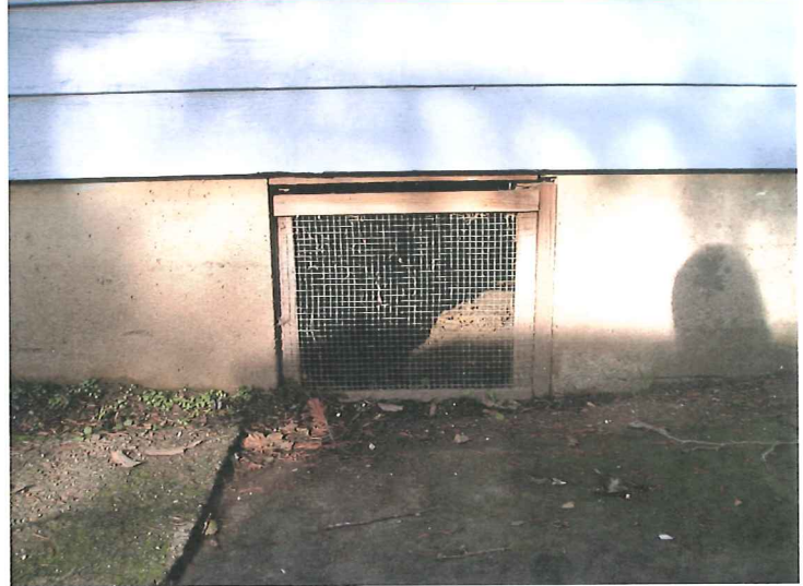
OPENING IN FOUNDATION (CRAWLSPACE ACCESS)
