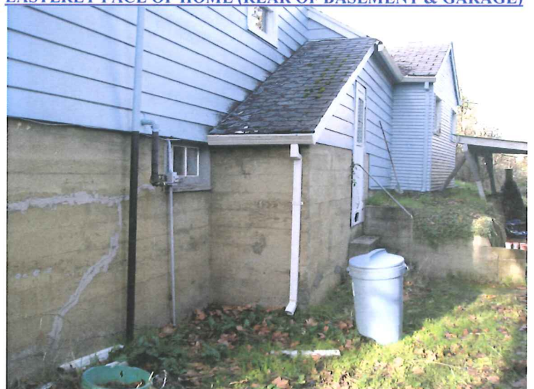
EASTERLY FACE OF HOME (REAR OF BASEMENT & GARAGE)
