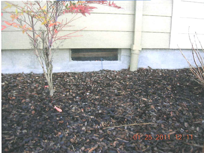
TYPICAL FOUNDATION VENT
