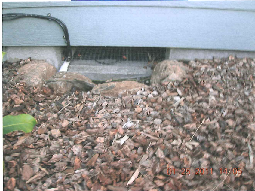
TYPICAL FOUNDATION VENT
