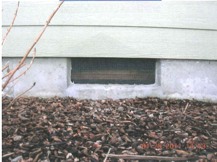
TYPICAL FOUNDATION VENT
