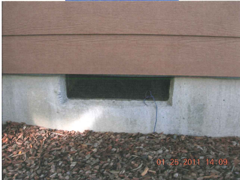
TYPICAL FOUNDATION VENT
