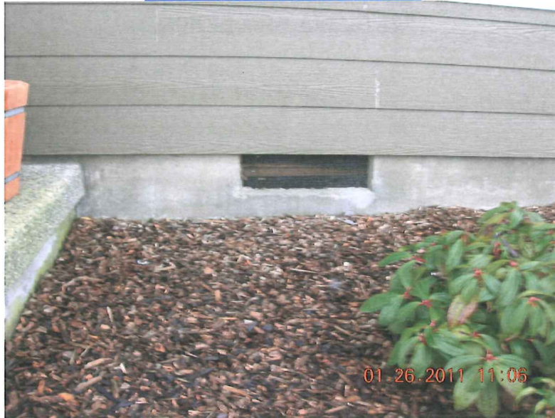
TYPICAL FOUNDATION VENT
