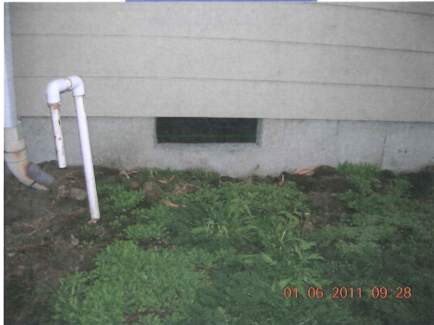
TYPICAL FOUNDATION VENT
