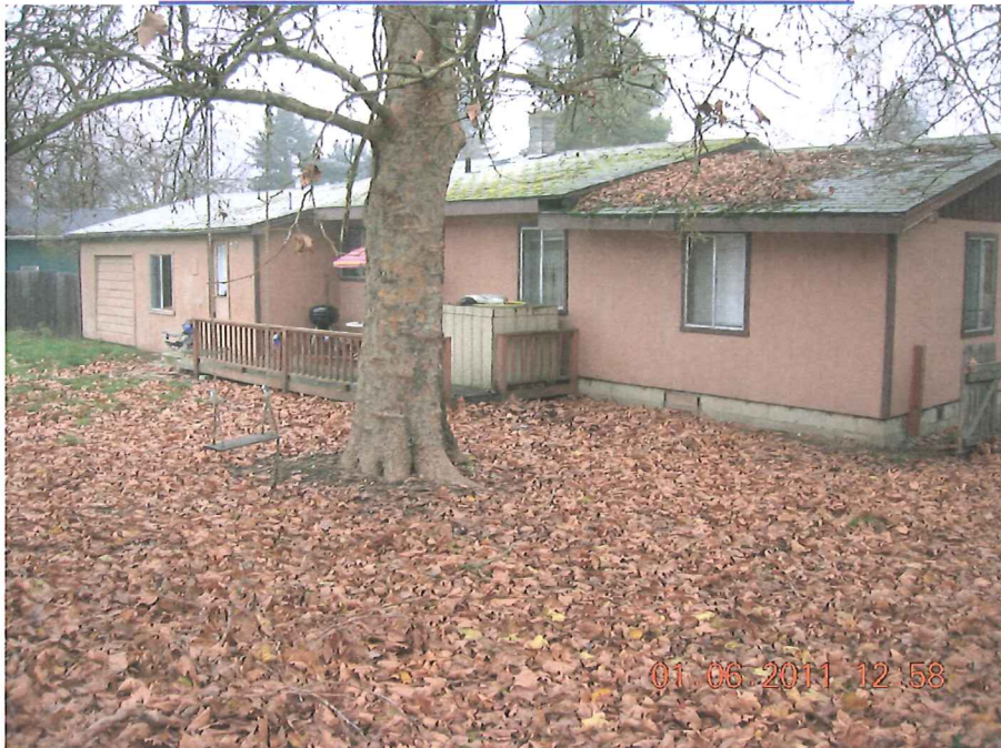
WEST FACE OF HOME (LOOKING NORTHERLY)
