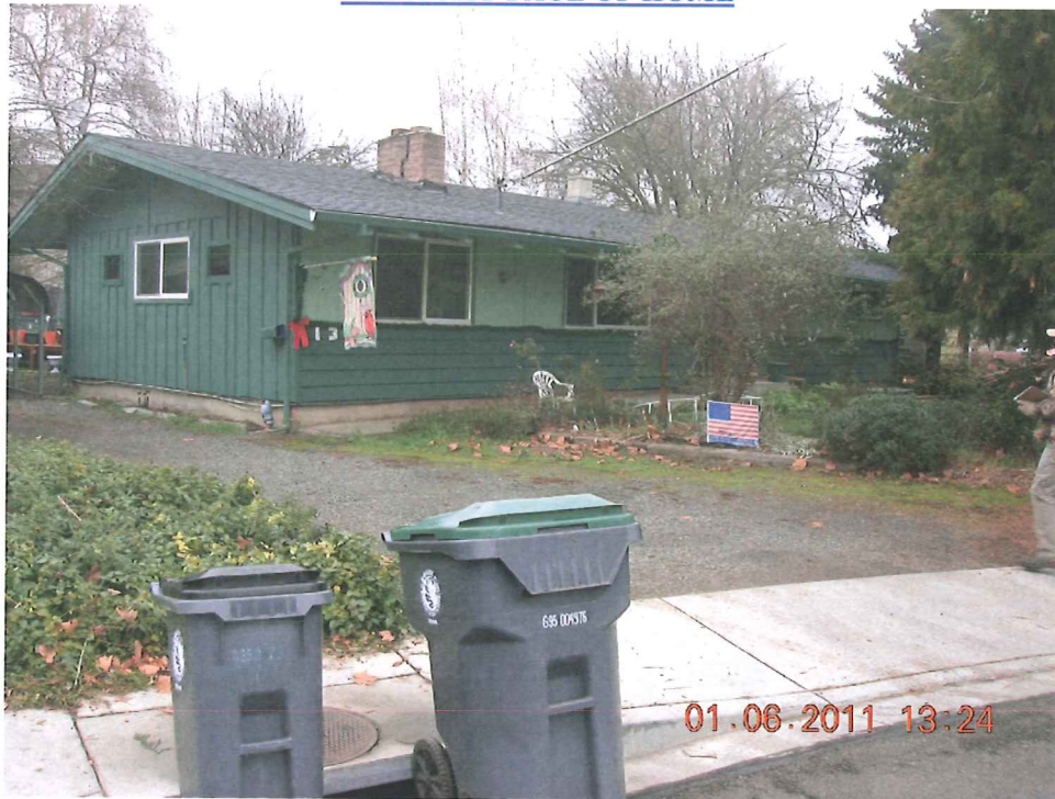
EASTERLY FACE OF HOME
