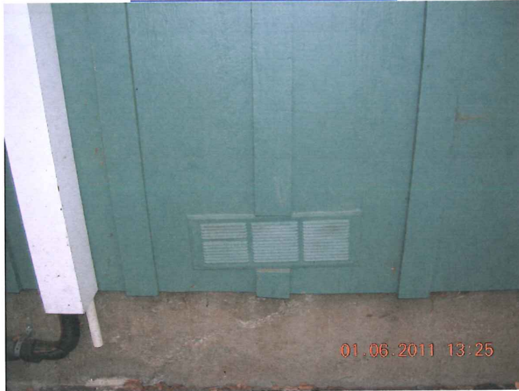
TYPICAL FOUNDATION VENT
