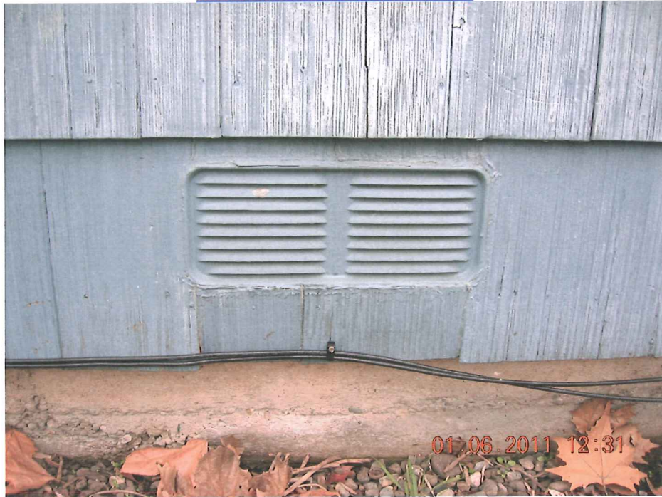
TYPICAL FOUNDATION VENT
