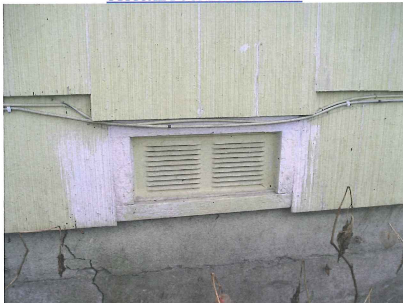
TYPICAL FOUNDATION VENT
