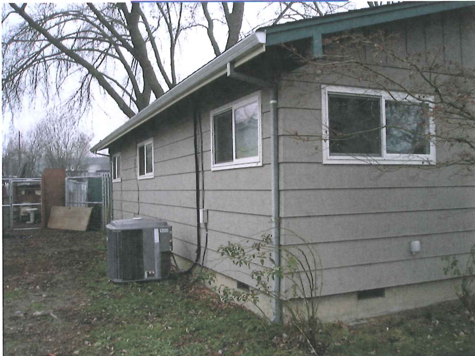
HEAT PUMP ON CONCRETE PAD
