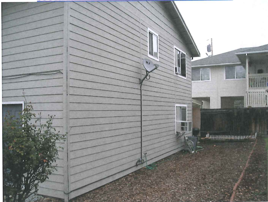
SOUTH FACE OF BUILDING (LOOKING EASTERLY)
