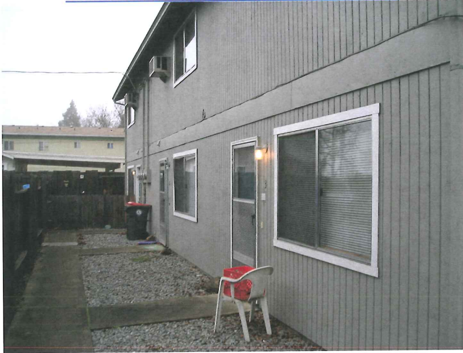
NORTH FACE OF BUILDING (LOOKING EASTERLY)
