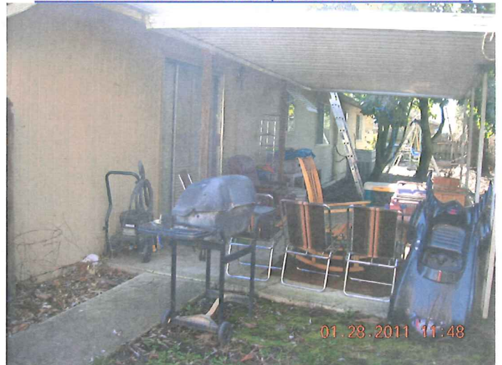
WESTERLY FACE OF HOME (LOOKING SOUTHERLY)
