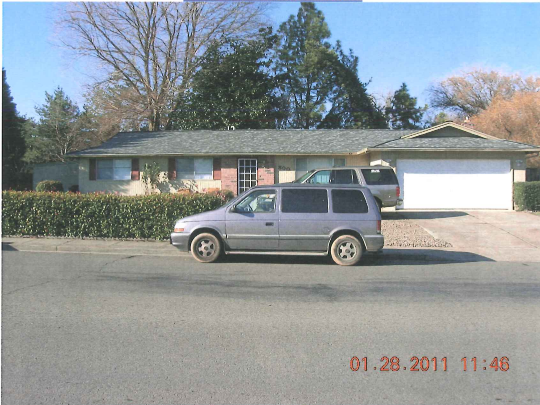
EASTERLY FACE OF HOME
