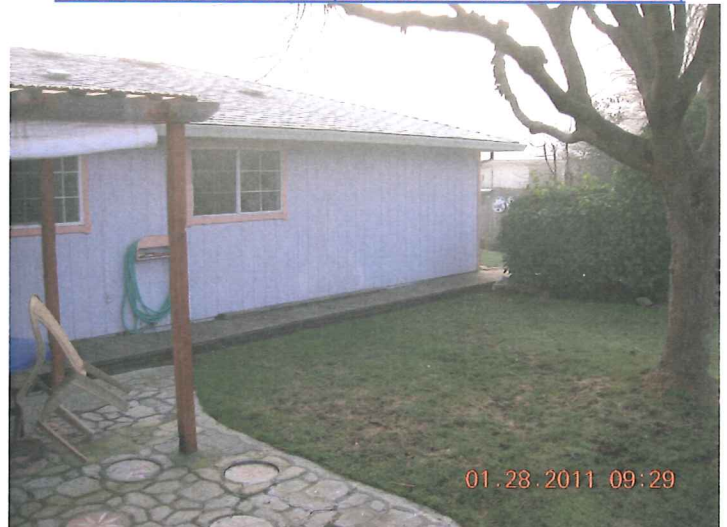
SOUTHWEST CORNER (LOOKING SOUTHEASTERLY)
