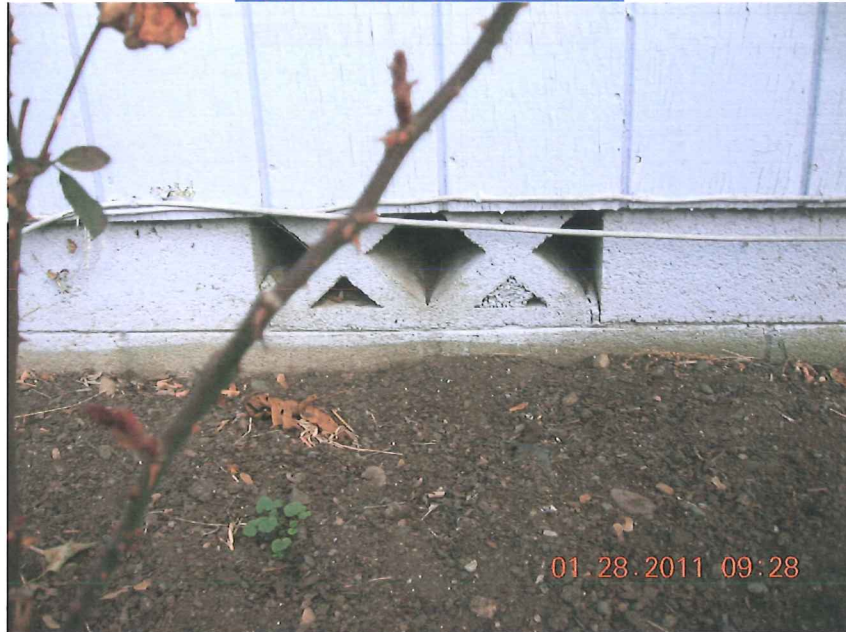
TYPICAL FOUNDATION VENT
