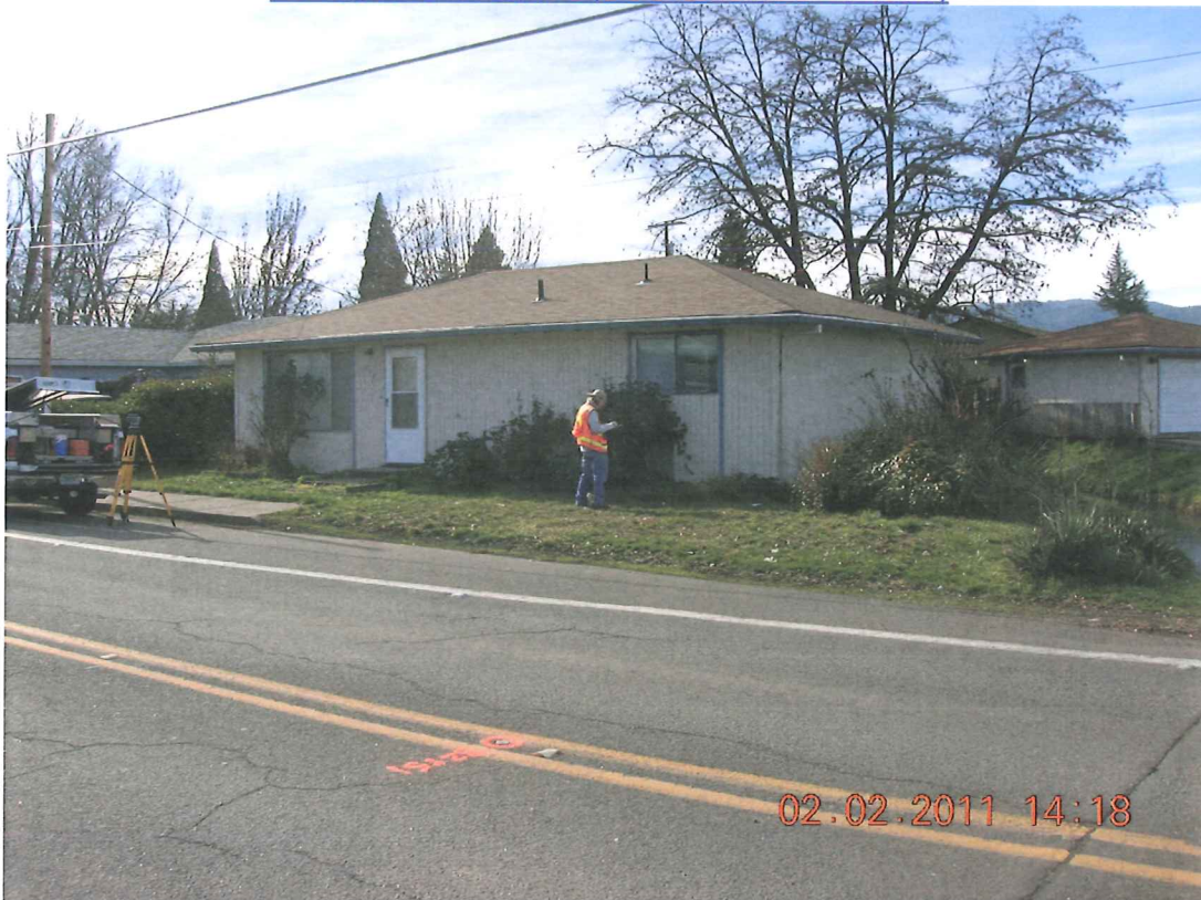
EAST FACE OF HOME (LOOKING SOUTHERLY)
