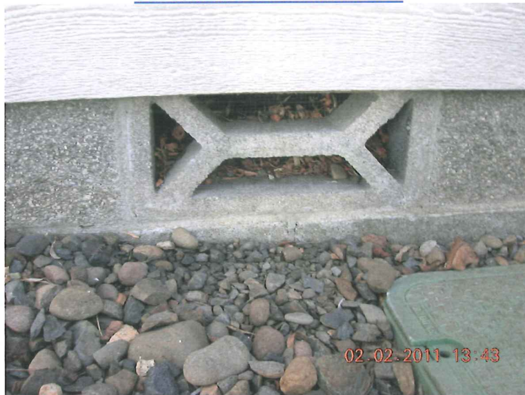
TYPICAL FOUNDATION VENT
