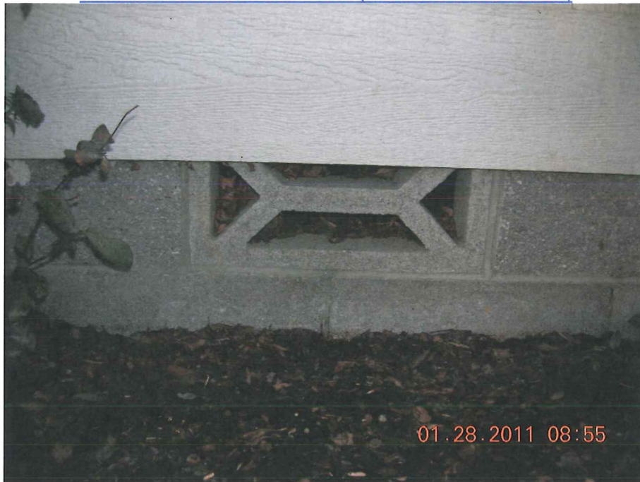
TYPICAL FOUNDATION VENT (DECORATIVE BLOCK)
