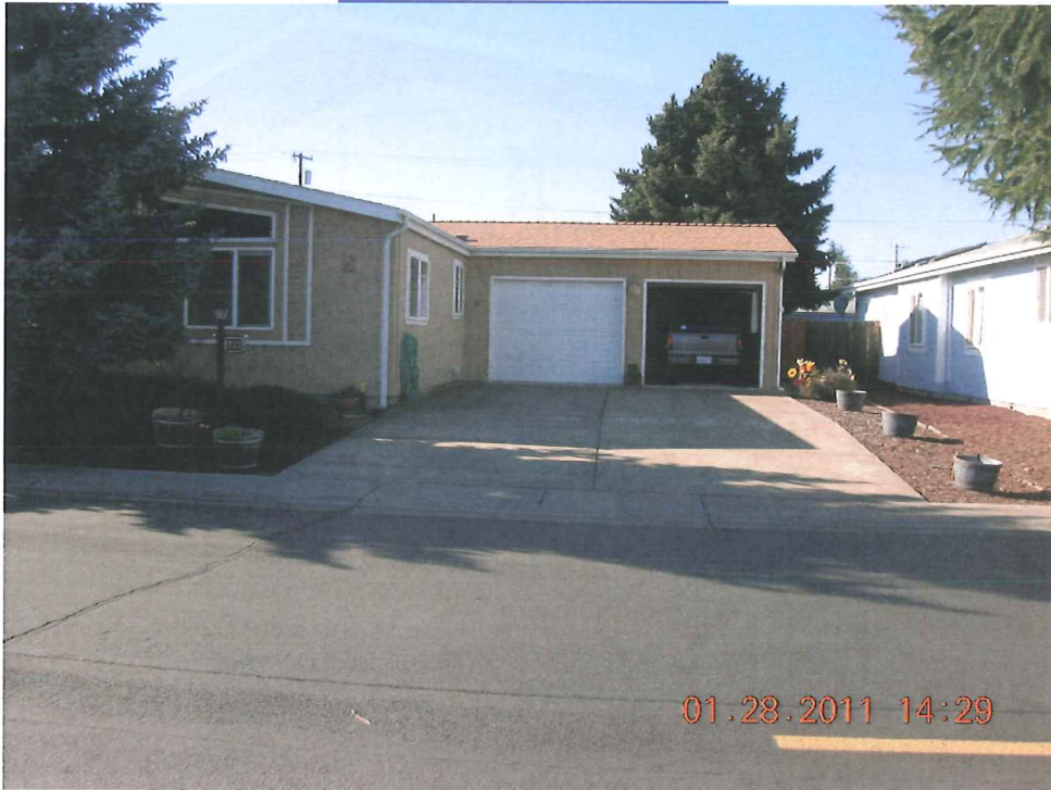
EASTERLY FACE OF HOME
