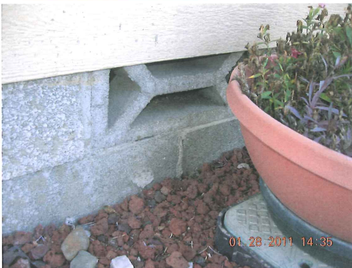
TYPICAL FOUNDATION VENT (DECORATIVE BLOCK)
