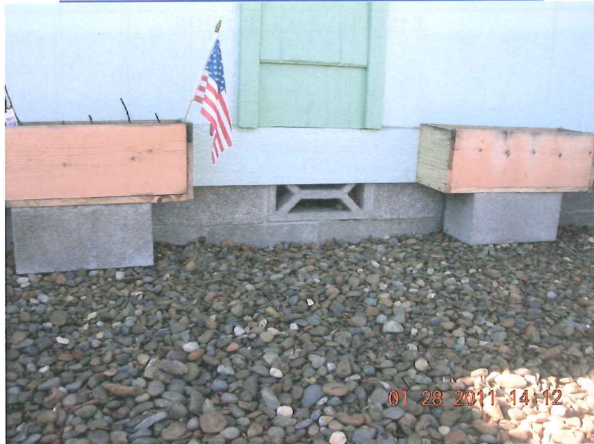
TYPICAL FOUNDATION VENT (DECORATIVE BLOCK)
