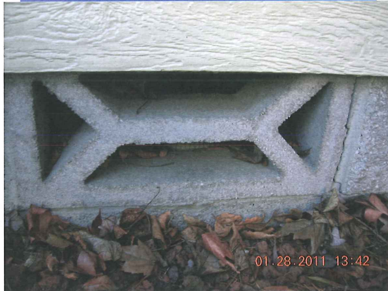
TYPICAL FOUNDATION VENT (DECORATIVE BLOCK)
