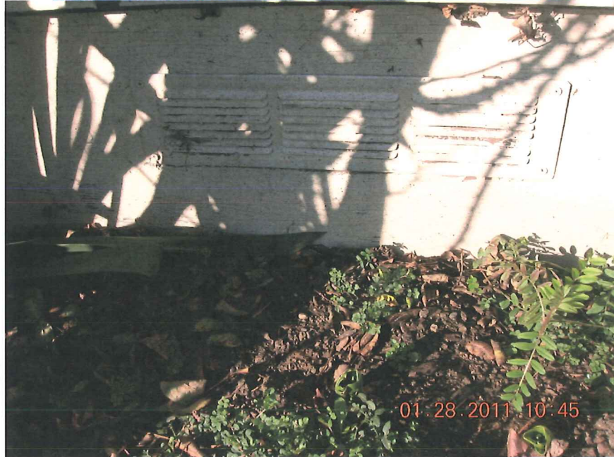
TYPICAL FOUNDATION VENT WITH LOUVERED COVER
