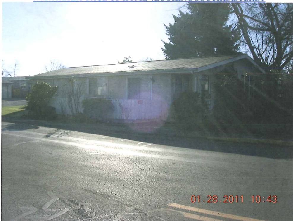
NORTHERLY FACE OF HOME (LOOKING SOUTHEASTERLY)
