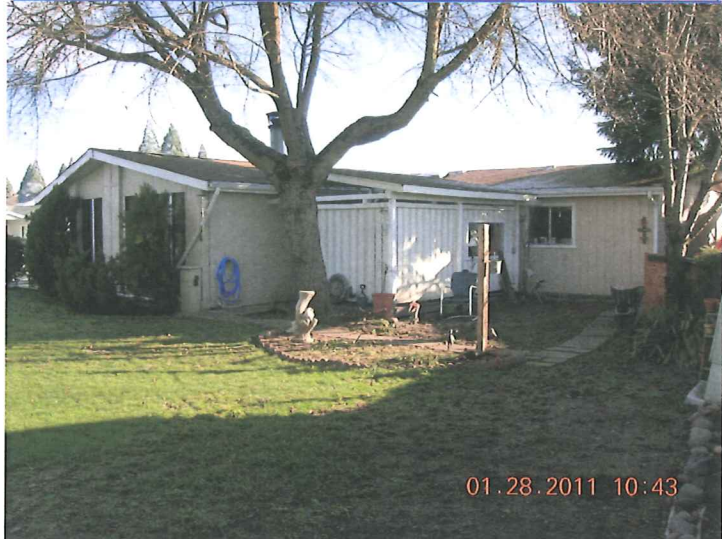
SOUTHERLY FACE OF HOME (LOOKING NORTHEASTERLY)
