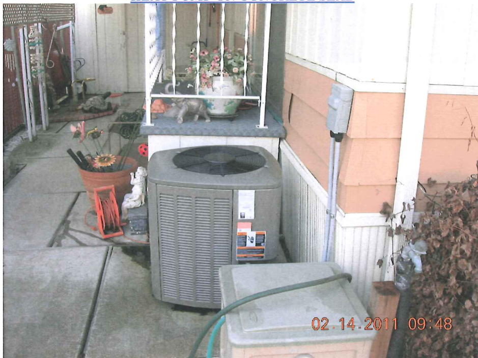
HEAT PUMP ON CONCRETE SLAB
