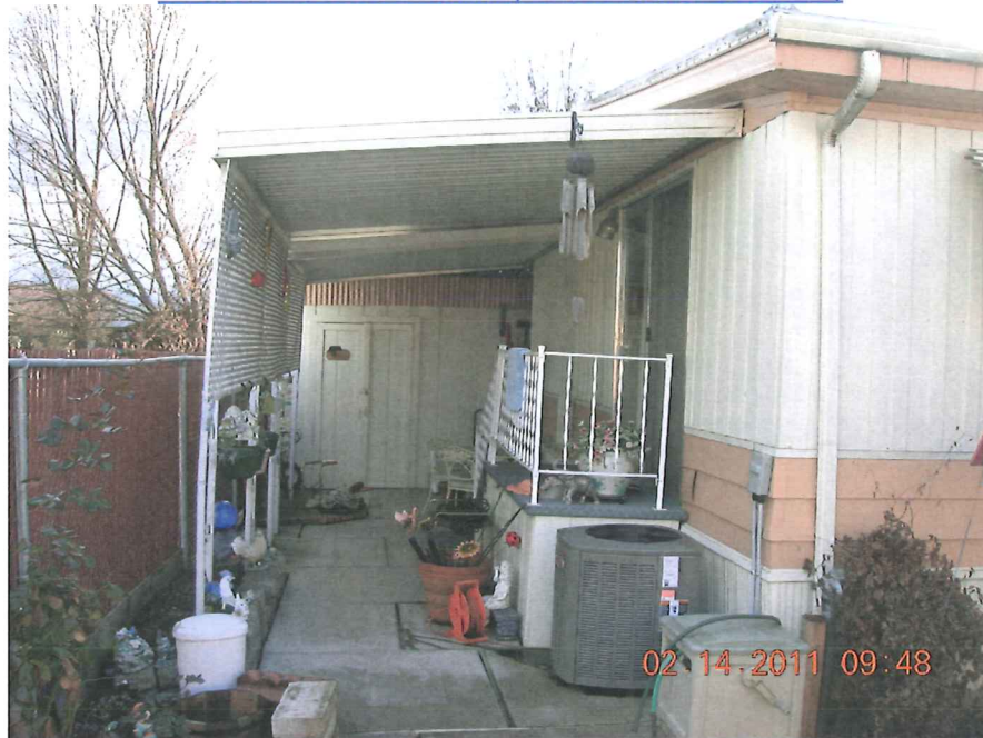
HEAT PUMP ON CONCRETE SLAB
