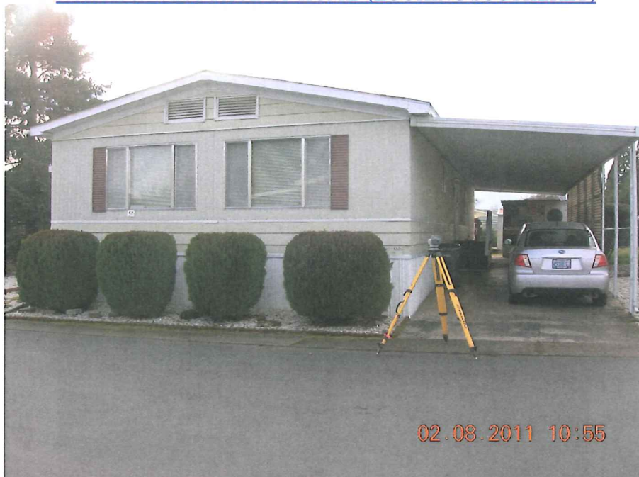
NORTH & WEST FACE OF HOME (LOOKING SOUTHERLY)
