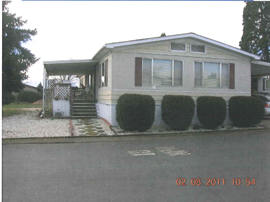
NORTH & EAST FACE OF HOME (LOOKING SOUTHERLY)
