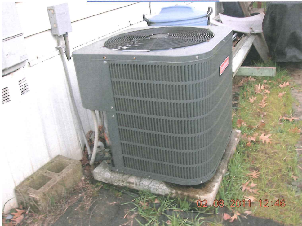
HEAT PUMP ON CONCRETE PAD
