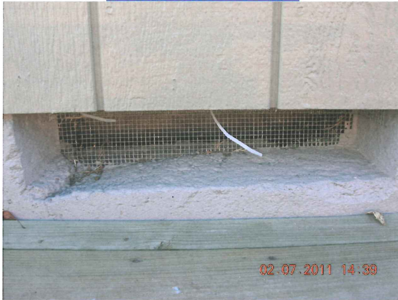
TYPICAL FOUNDATION VENT
