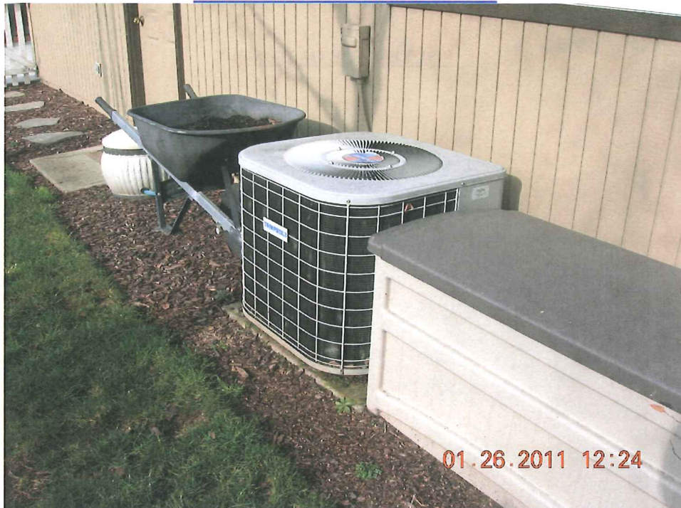
HEAT PUMP ON CONCRETE PAD
