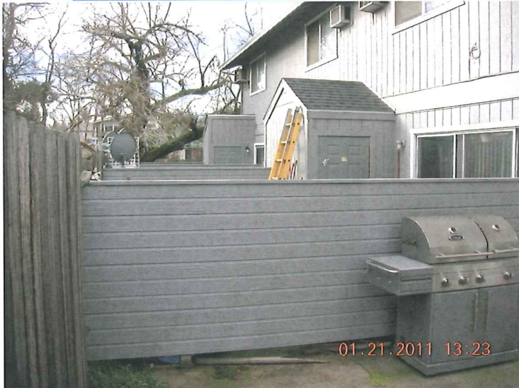
SOUTH FACE OF (LOOKING WESTERLY)
