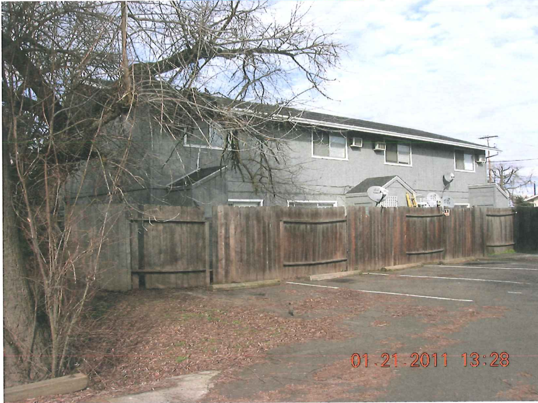
SOUTH FACE OF BUILDING
