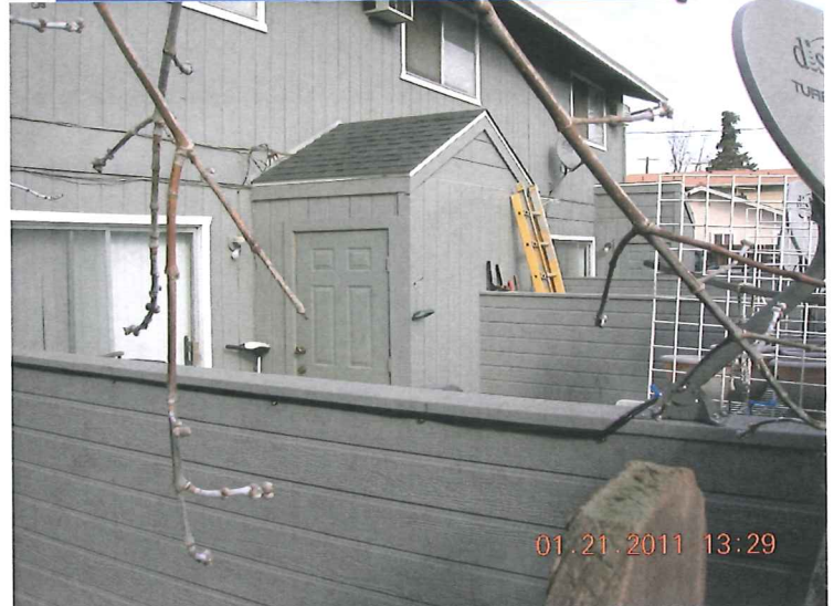
SOUTH FACE OF BUILDING (LOOKING EASTERLY)
