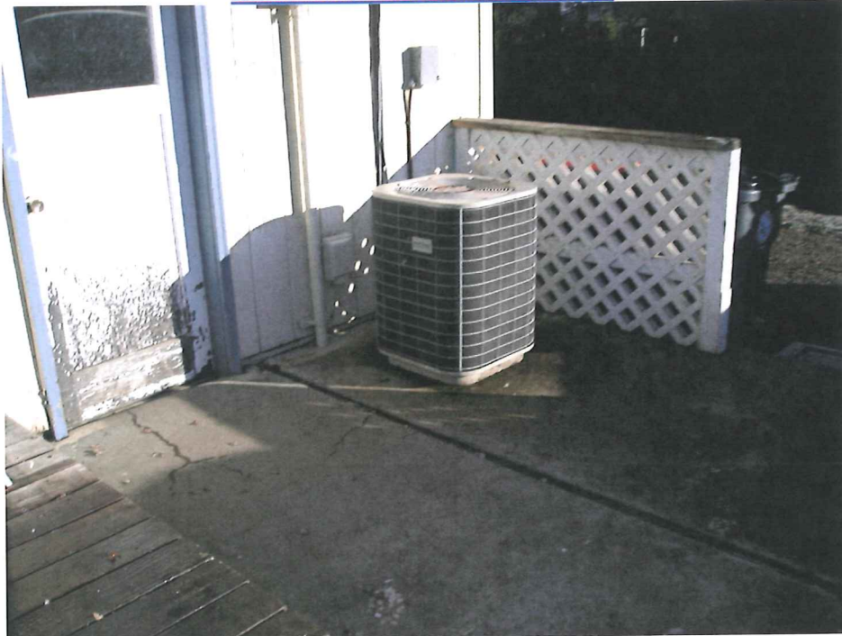
HEAT PUMP ON CONCRETE PAD
