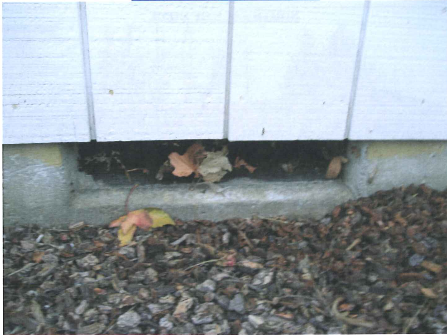
TYPICAL FOUNDATION VENT
