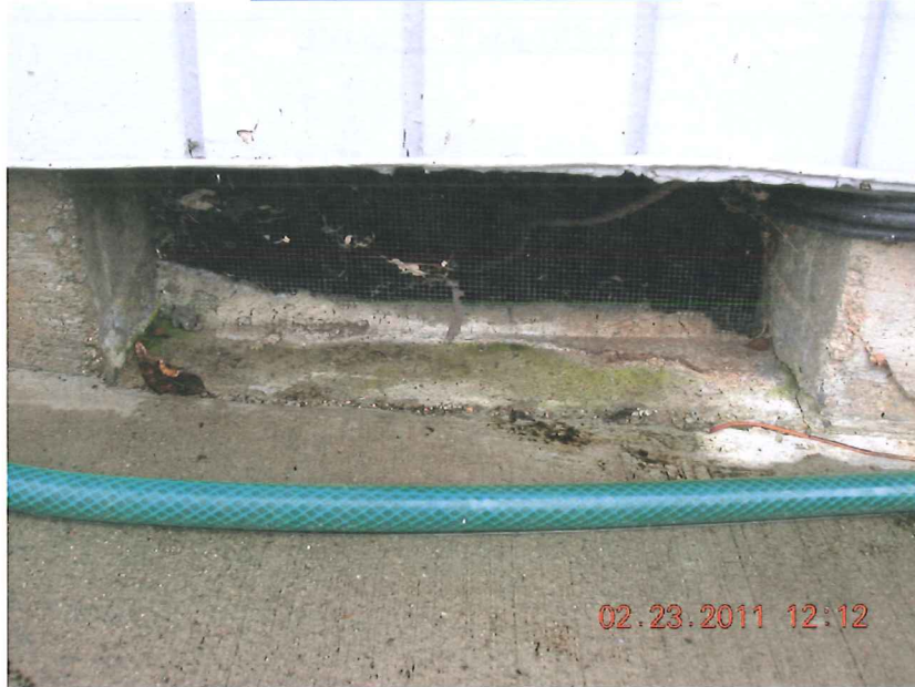
TYPICAL FOUNDATION VENT
