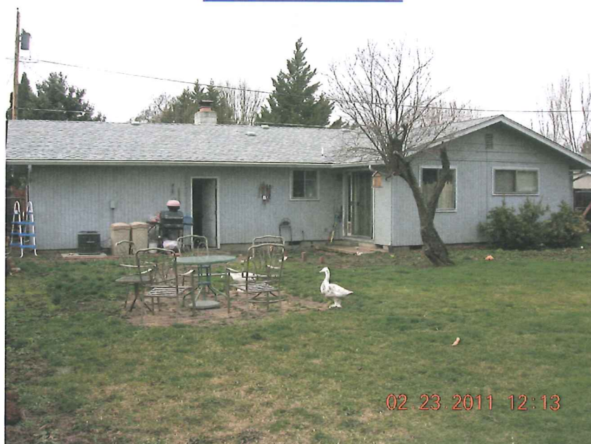
EAST FACE OF HOME
