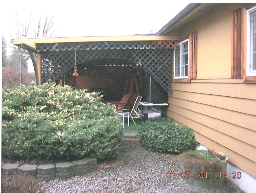
EAST FACE OF HOME (LOOKING SOUTHERLY)
