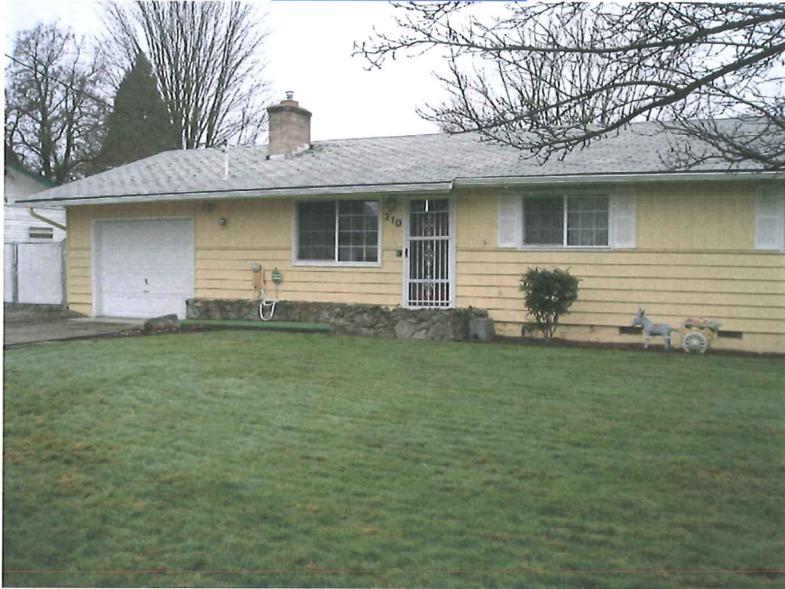
EAST FACE OF HOME
