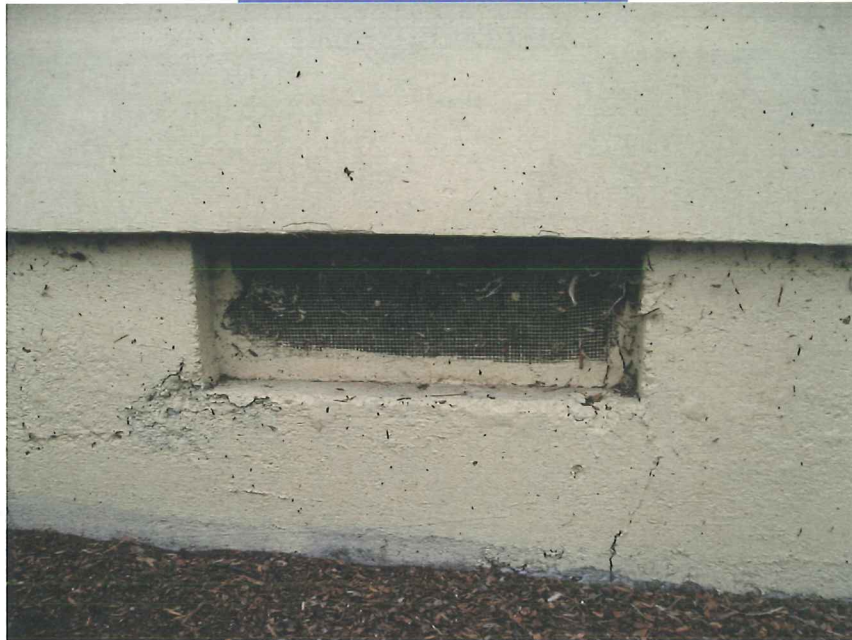
TYPICAL FOUNDATION VENT
