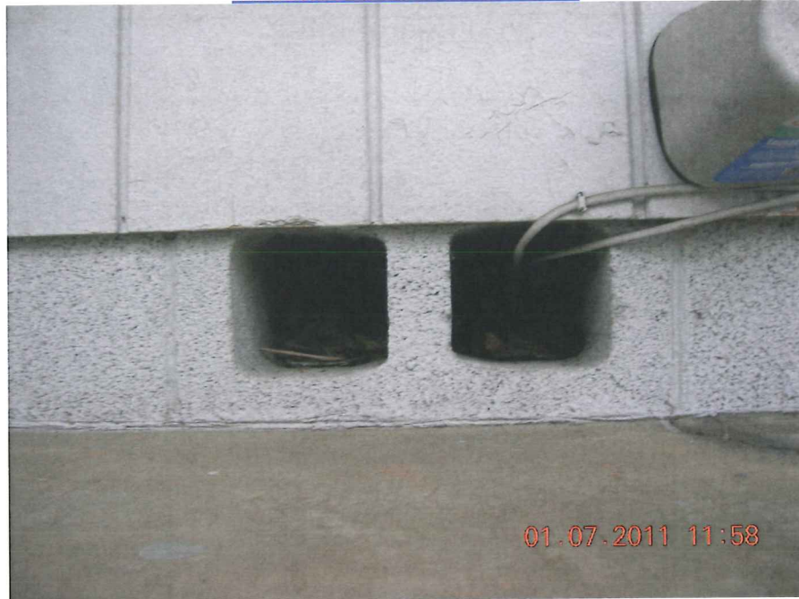
TYPICAL FOUNDATION VENT
