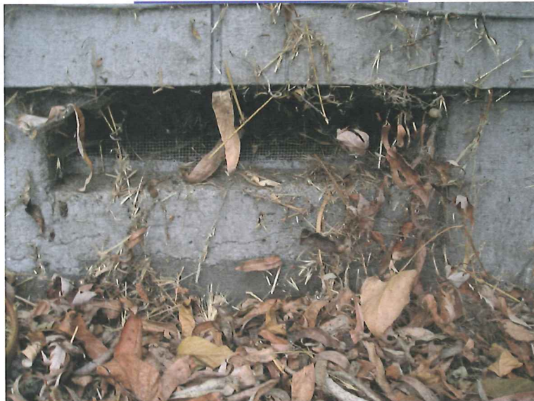
TYPICAL FOUNDATION VENT
