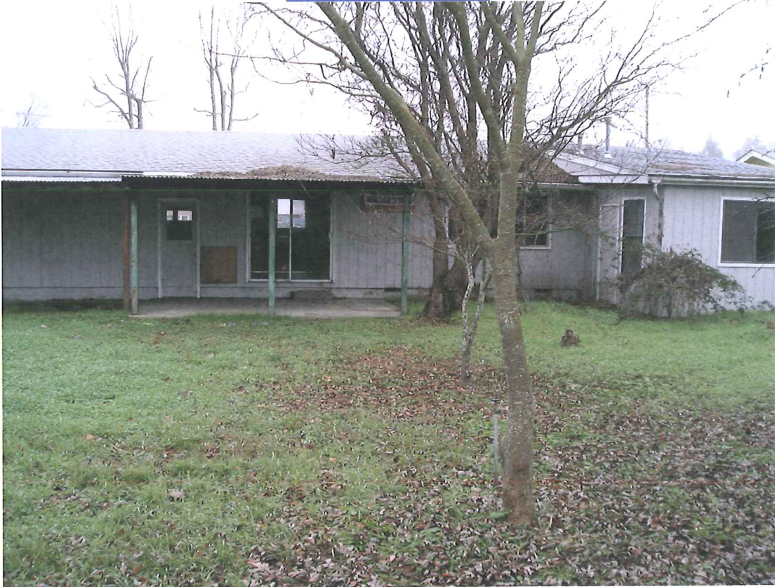
WEST FACE OF HOME
