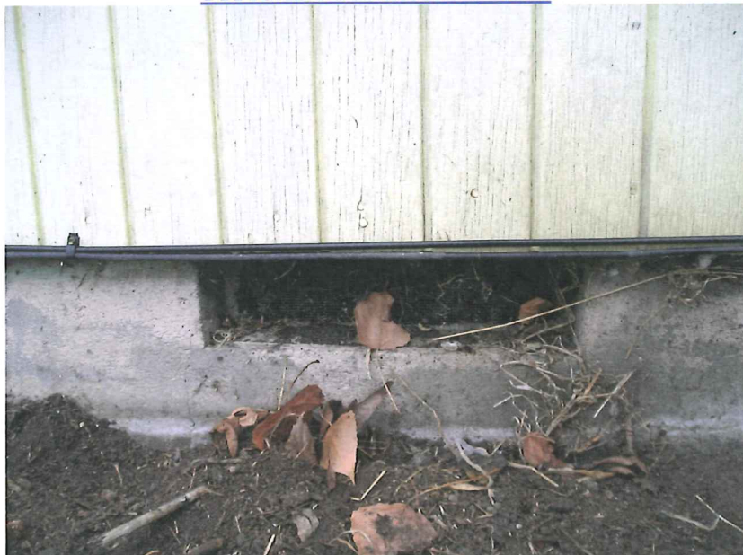
TYPICAL FOUNDATION VENT
