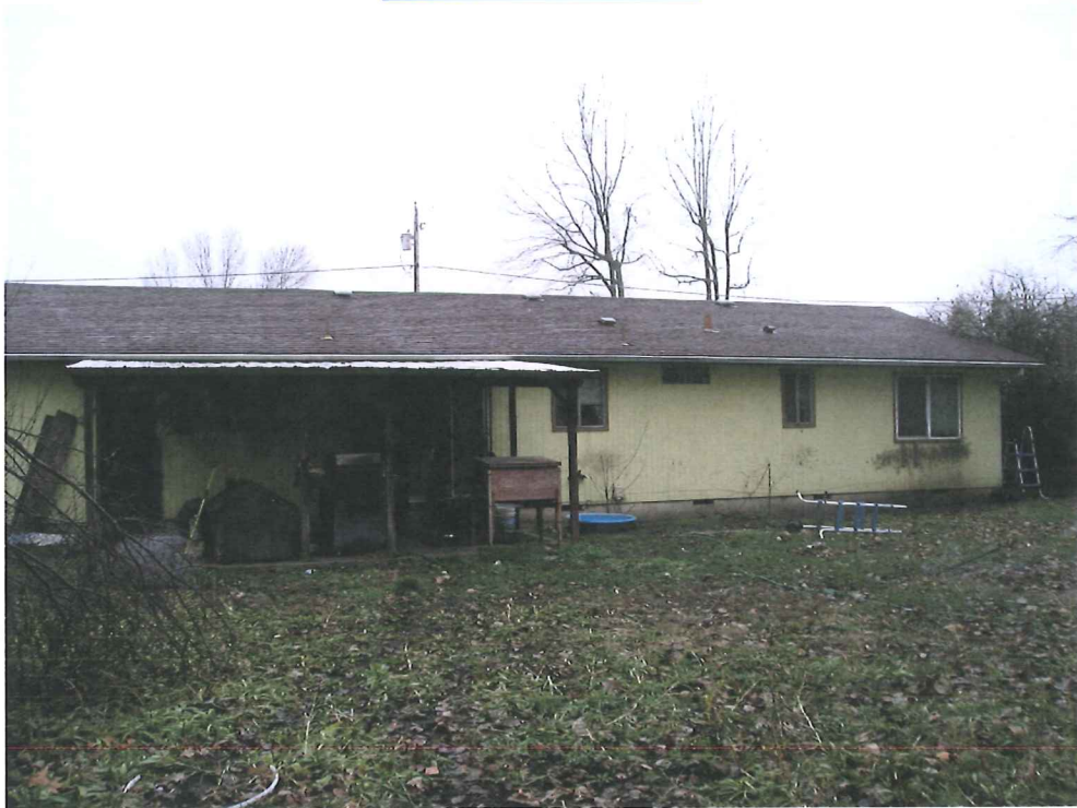
WEST FACE OF HOME
