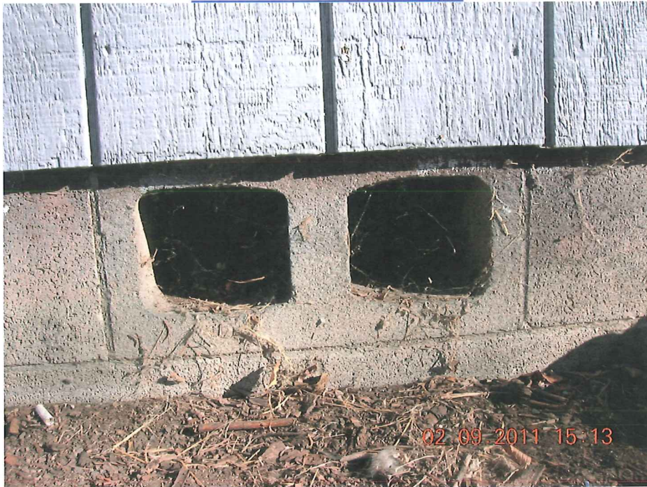
TYPICAL FOUNDATION VENT
