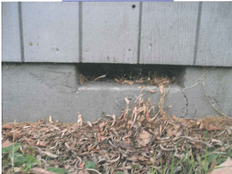
TYPICAL FOUNDATION VENT
