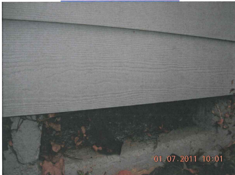
TYPICAL FOUNDATION VENT
