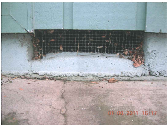
TYPICAL FOUNDATION VENT
