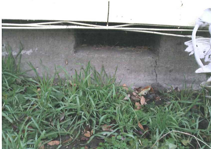
TYPICAL FOUNDATION VENT
