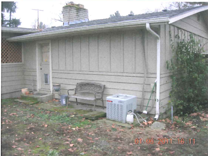
EASTERLY FACE OF GARAGE AND HEAT PUMP
