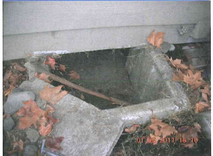
CRAWLSPACE ACCESS (AT EASTERLY FACE OF HOME)
