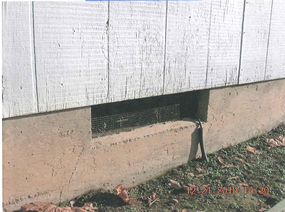
TYPICAL FOUNDATION VENT
