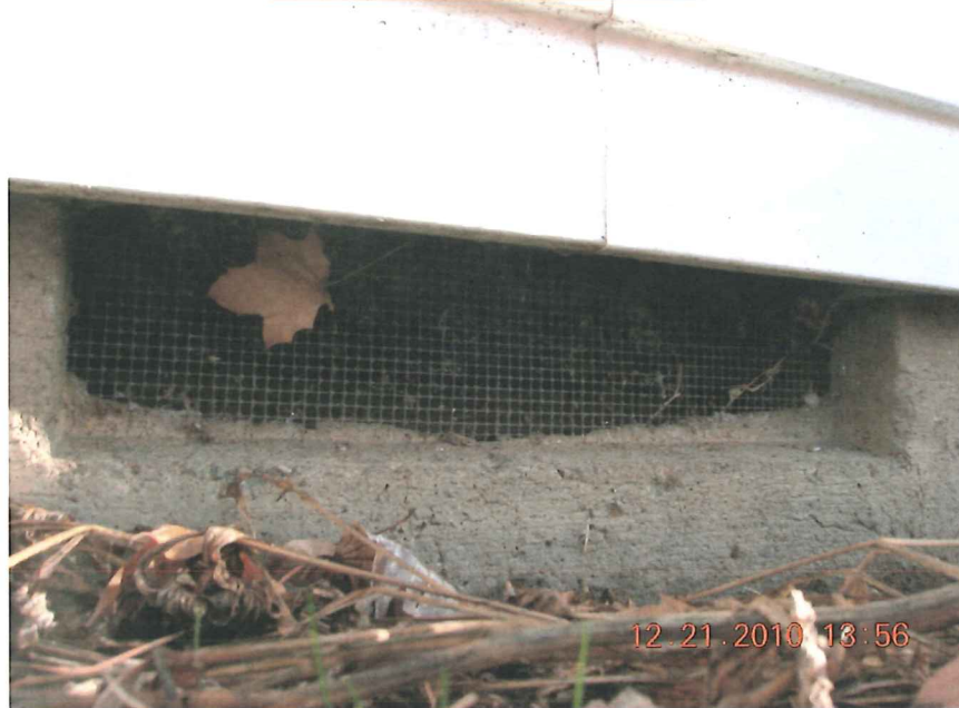
TYPICAL FOUNDATION VENT
