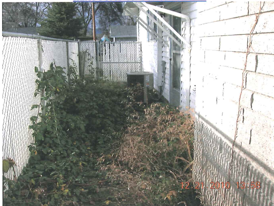
HEAT PUMP ON CONCRETE PAD
