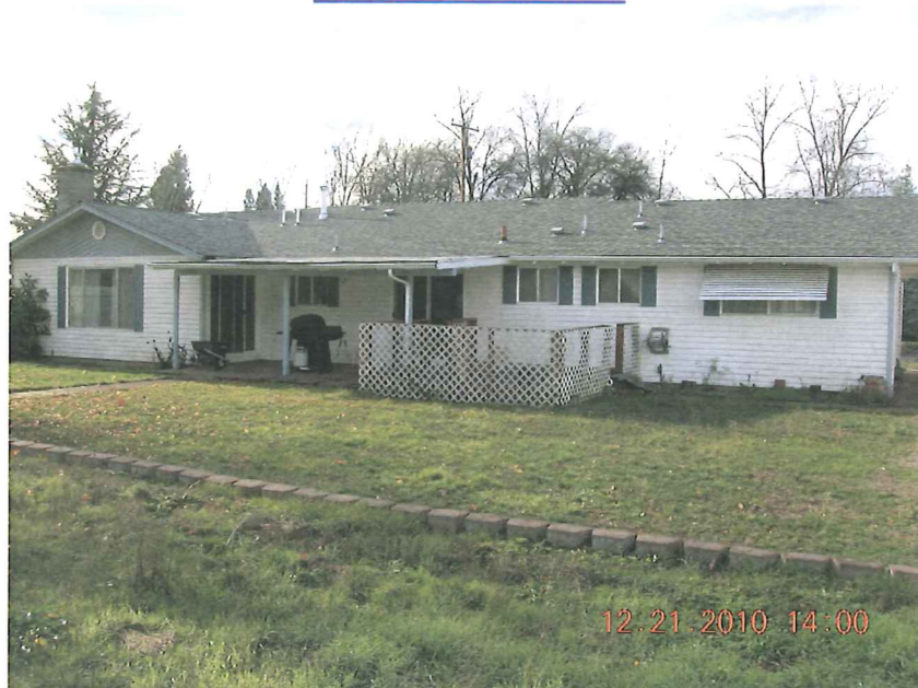
EAST FACE OF HOME
