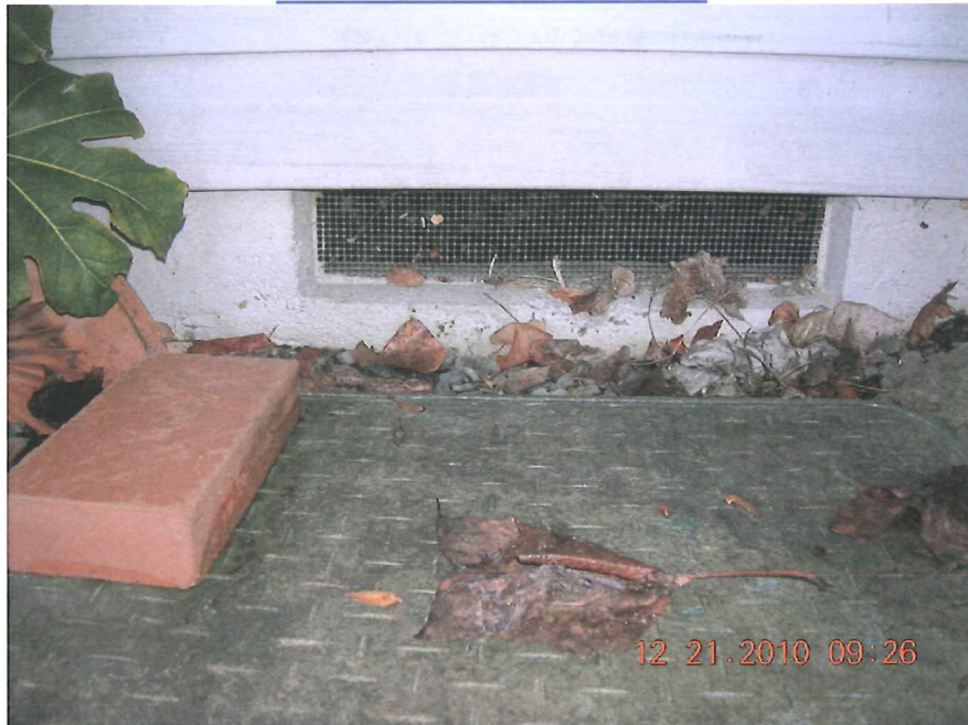
TYPICAL FOUNDATION VENT
