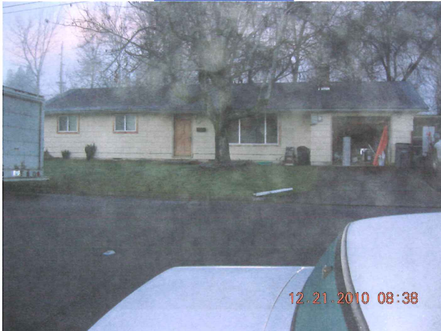
EAST FACE OF HOME
