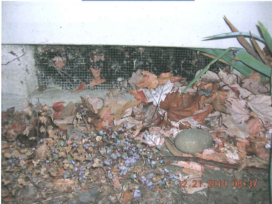
TYPICAL FOUNDATION VENT
