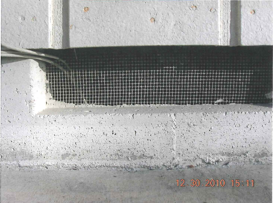
TYPICAL FOUNDATION VENT
