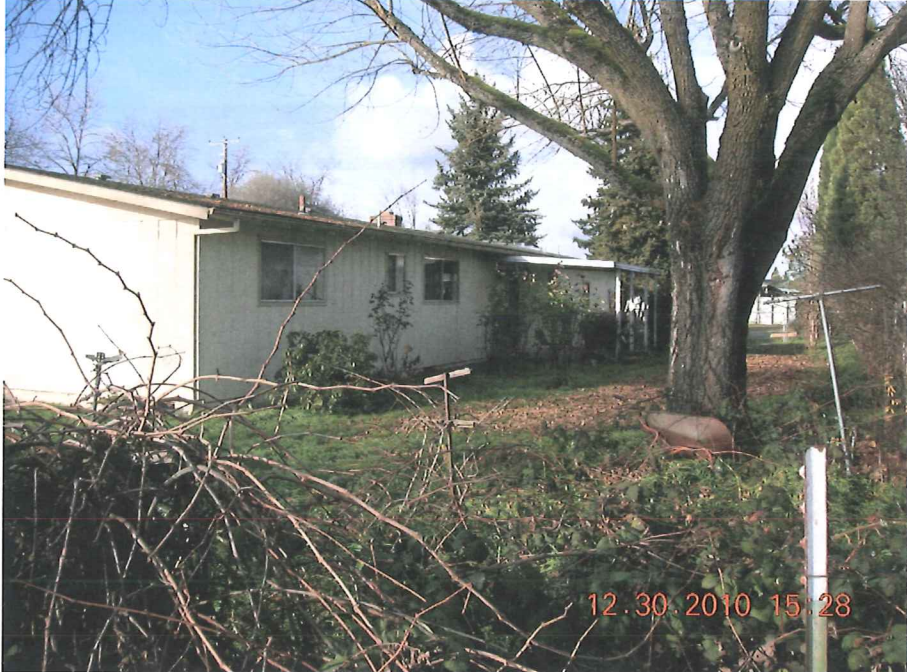
EAST FACE OF HOME (LOOKING NORTHERLY)
