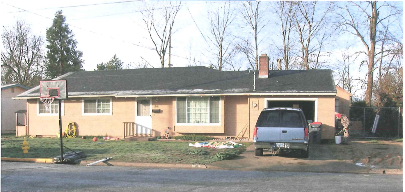
EASTERLY FACE OF HOME
