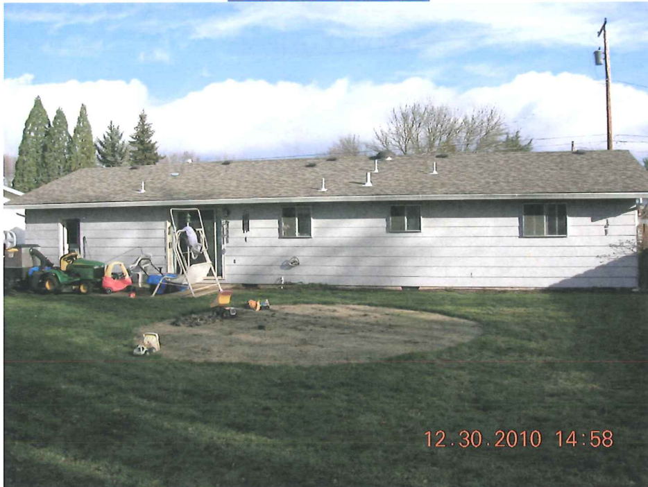
WEST FACE OF HOME
